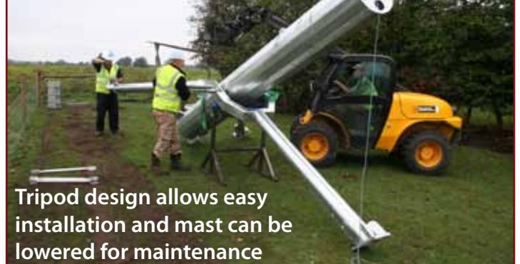
Tripod design allows easy installation and mast can be lowered for maintenance
