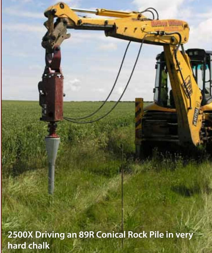
2500X Driving an 89R Conical Rock Pile in very hard chalk
